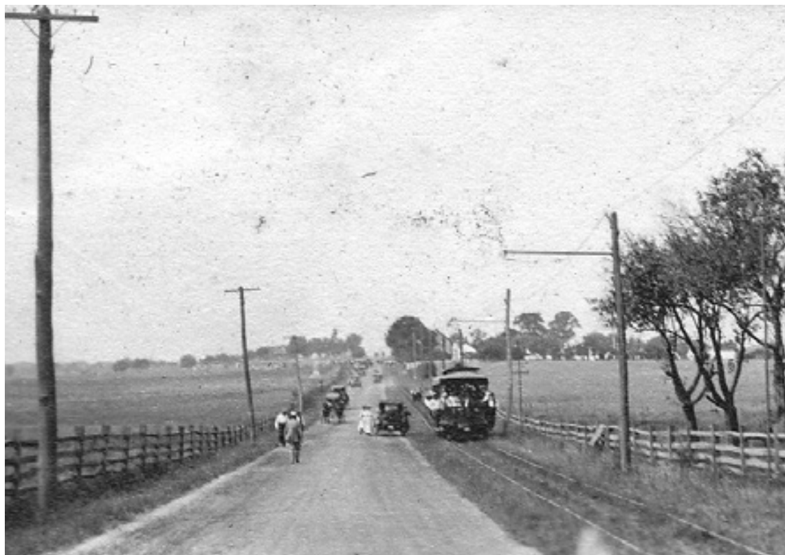
Visitors to the 1913 reunion walk and ride along Old Emmitsburg Road near the 'Peach Grove' on the battlefield. Note the old trolley line that used to run along the road.
