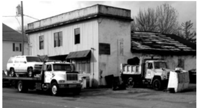
Old East End Garage was razed to make room for a new Dollar General Store, construction for which will begin in early 2015.
