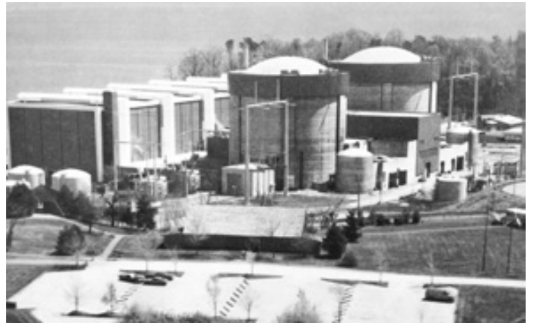
The Calvert Cliffs Nuclear Power Plant, located on the western shore of the Chesapeake Bay in Calvert County, Maryland, produces 1/3rd of all the electricity used in Maryland with absolutely zero carbon or any global warming atmospheric emissions. The two reactors went on line in 1975 and 1977 at a total cost $766 million. In 2009, Calvert Cliffs set a world record by operating for 692 days before shutting down to be refueled.
