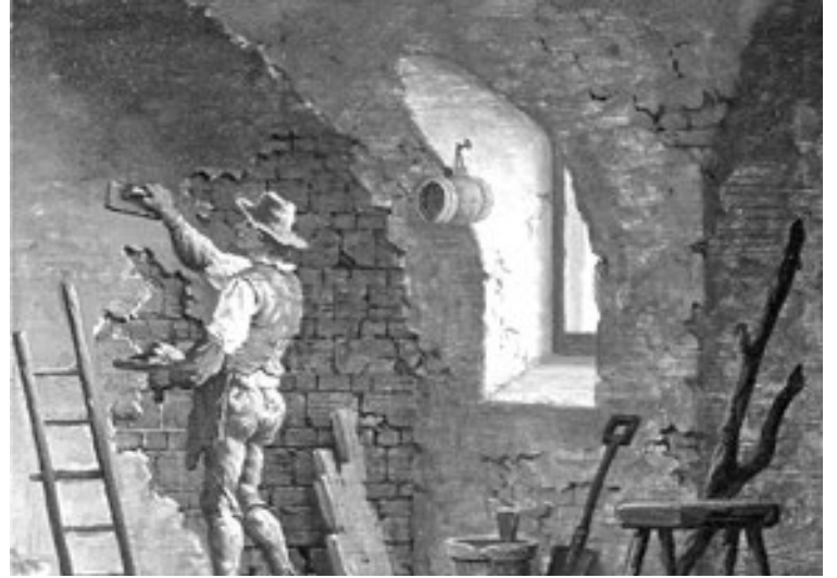
Plaster at work in the early 1800s. Plaster not only provided an esthetic appearance, but in homes made of wood, served to seal out drafts coming through the walls.
