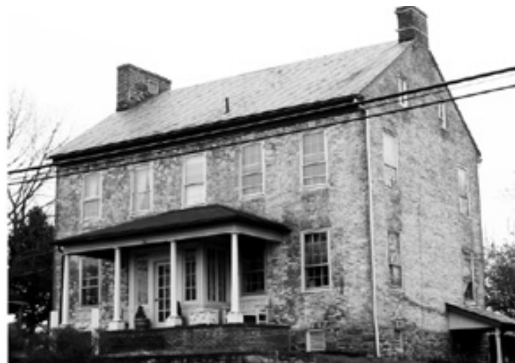
The Ludwick Rudisel Tannery House, also known as Motter Place, was built around 1807.
