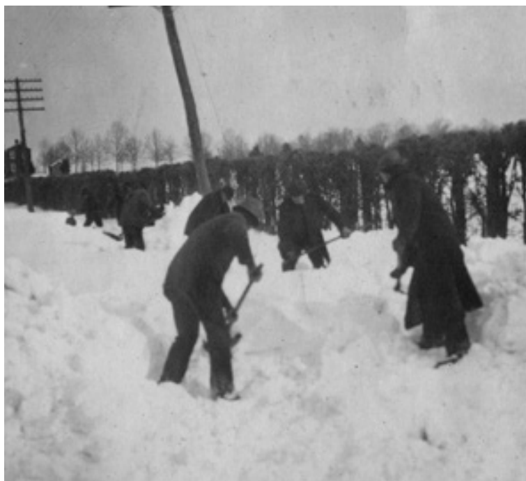
If you thought shoveling your driveway was hard work, try shoveling a road by hand!
